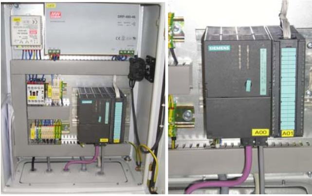
Fig. 9: Position of S7-300 and SM-331 in the electrical case
